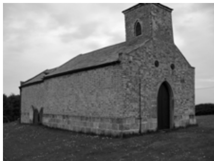
Ruston Parva showing the windowless north wall. Unusually for a C of E church there is a date stone near the door.
