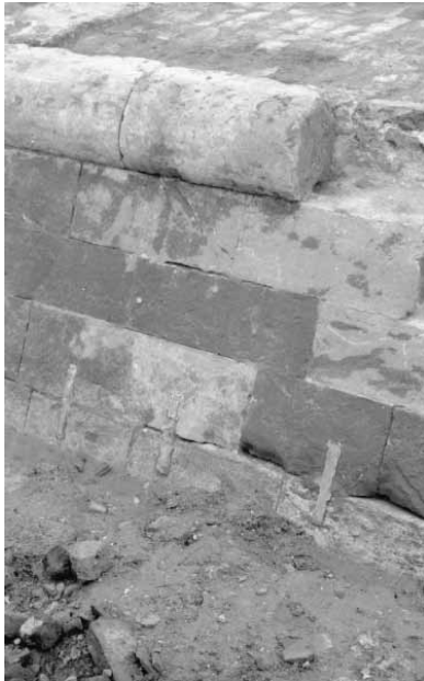
Humber wall, top of stone facing, lead tie-pins
