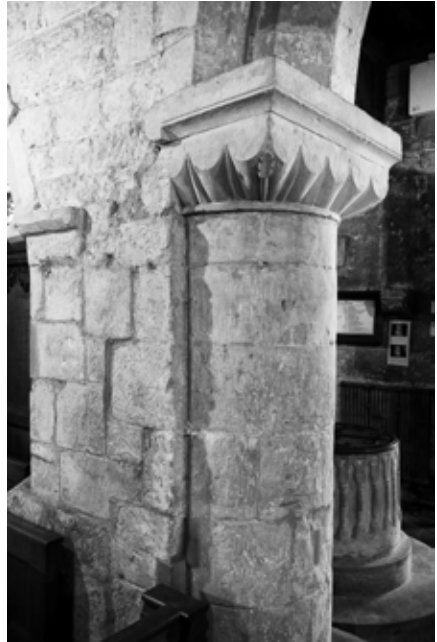
Norman pillar and capital in nave arcade.
