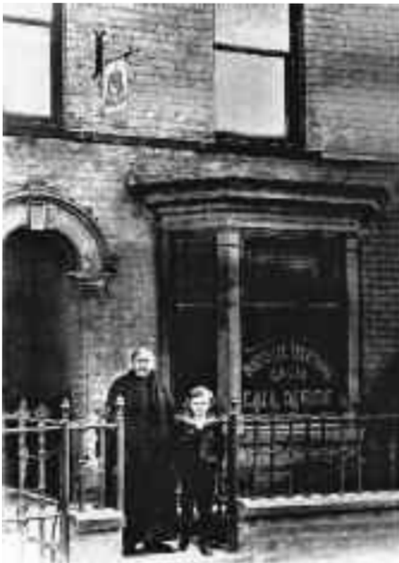
National Telephones, Kirkella Exchange
