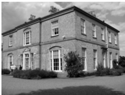
The west and south elevations
