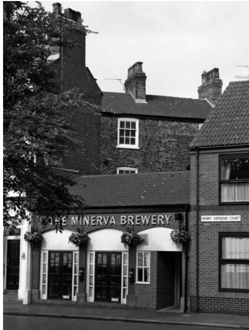
The brewery replaced the vaults and the old vaults roofline can be seen in the Minerva gable
